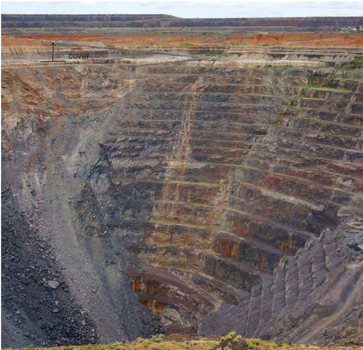
Figure 3.38. Photograph of the Ernest Henry pit looking to the south, showing the position of the Proterozoic unconformity.
