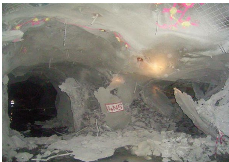
Figure 9. Example of where the vertical stress concentrations point loaded a drawpoint area causing the apex pillars to fail and the drawpoint becoming inaccessible.
