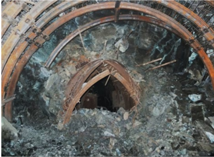
Figure 5. Example of squeezing ground conditions experienced at Cassier Mine in Canada, ultimately contributing to its premature closure.
